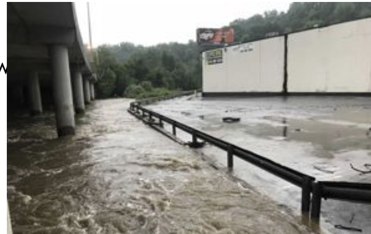
Severe flooding along the Jones Falls River in 2018
