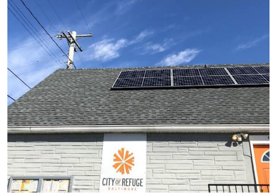
Solar Installation Complete (Jan 2021)
